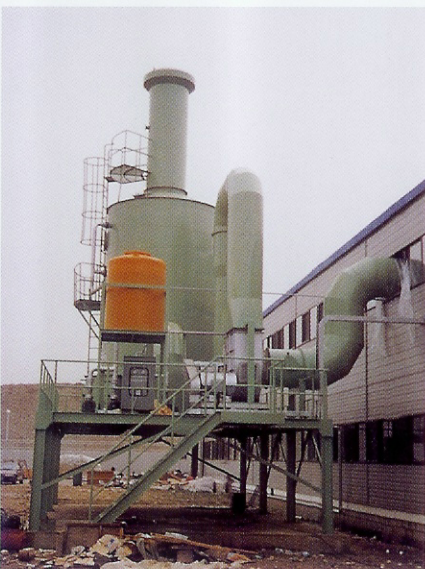
▲화학장치용 Scrubber(700 \text{m}^3/\text{min} )
