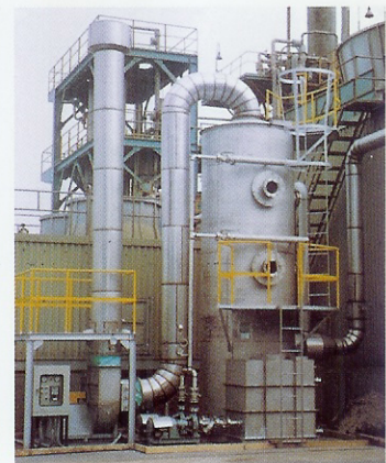
▲화학장치용 Packing Tower(320m 3 /min)
