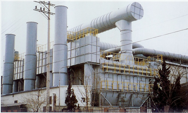
▲Air-Pulse Type Bag Filter(1,800m 3 /min)
