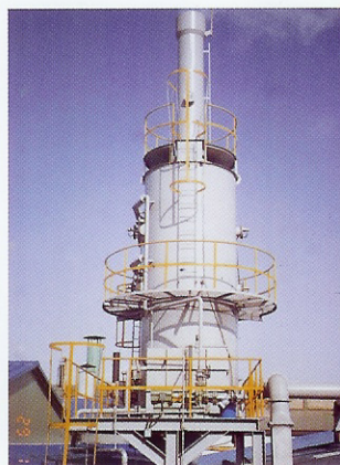
▲텐타기용 Packing Tower(280m 3 /min)
