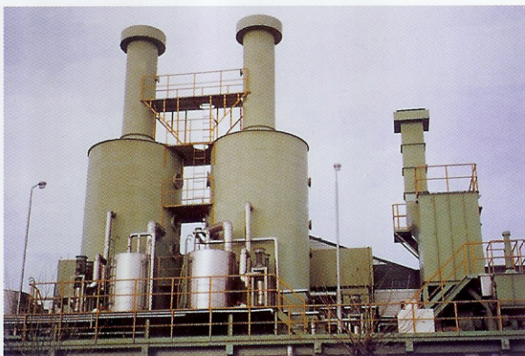
▲화학장치용 FRP Packing Tower(550m 3 /min×27l)
