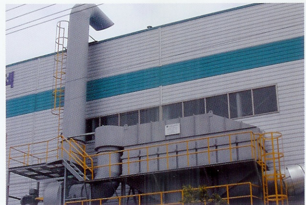
▲Oil Mist 제거설비(600m³/min)
