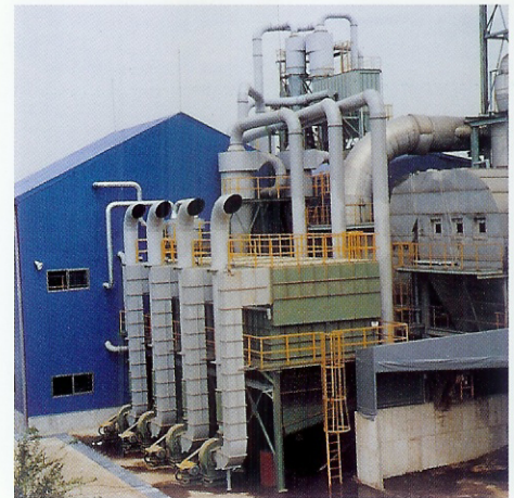
▲ Jet-Pulse Type Bag Filter(1,330m³/min)
