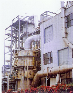
▲화학장치용 Packing Tower(900m 3 /min)
