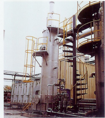
▲Impinzet Scrubber(450m 3 /min)
