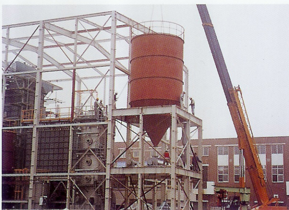
▲소각로용 Bagfilter + scrubber(500m 3 /min×27l)
