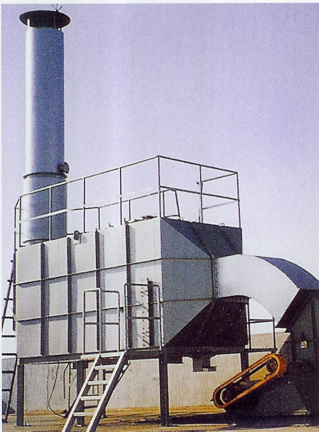
▲도장설비용 Active Carbon Tower(700m³/min)
