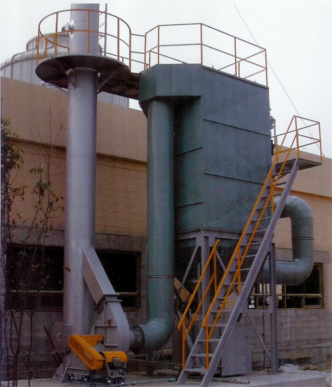
▲보일러용 Air-Pulse Bag Filter(300m 3 /min)
